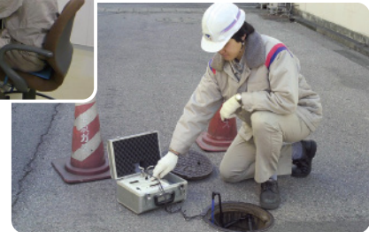
▲ 導管の電気防食評価試験 Field test of cathodic protection on pipeline
